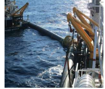
TRNC Water Pipeline (HDPE Pipeline)
