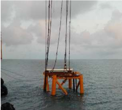
CPOC Block B17 (Jacket & Topside)
