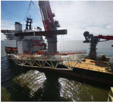
Petronas Baram (Bridge Replacement)
