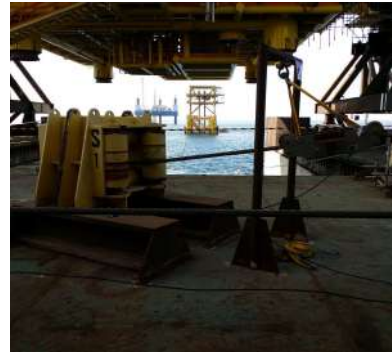
Petronas Turkmenistan (3 Topsides Floatovers)
