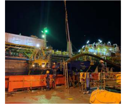
Petronas Jitang (FPSO Ledang Relocation)
